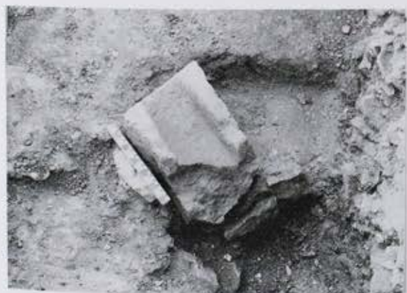
Fig 4.31 Drain: channel stone found in external area east of chapel N2 and north of chapel B1, Sq 3/73, 1969
